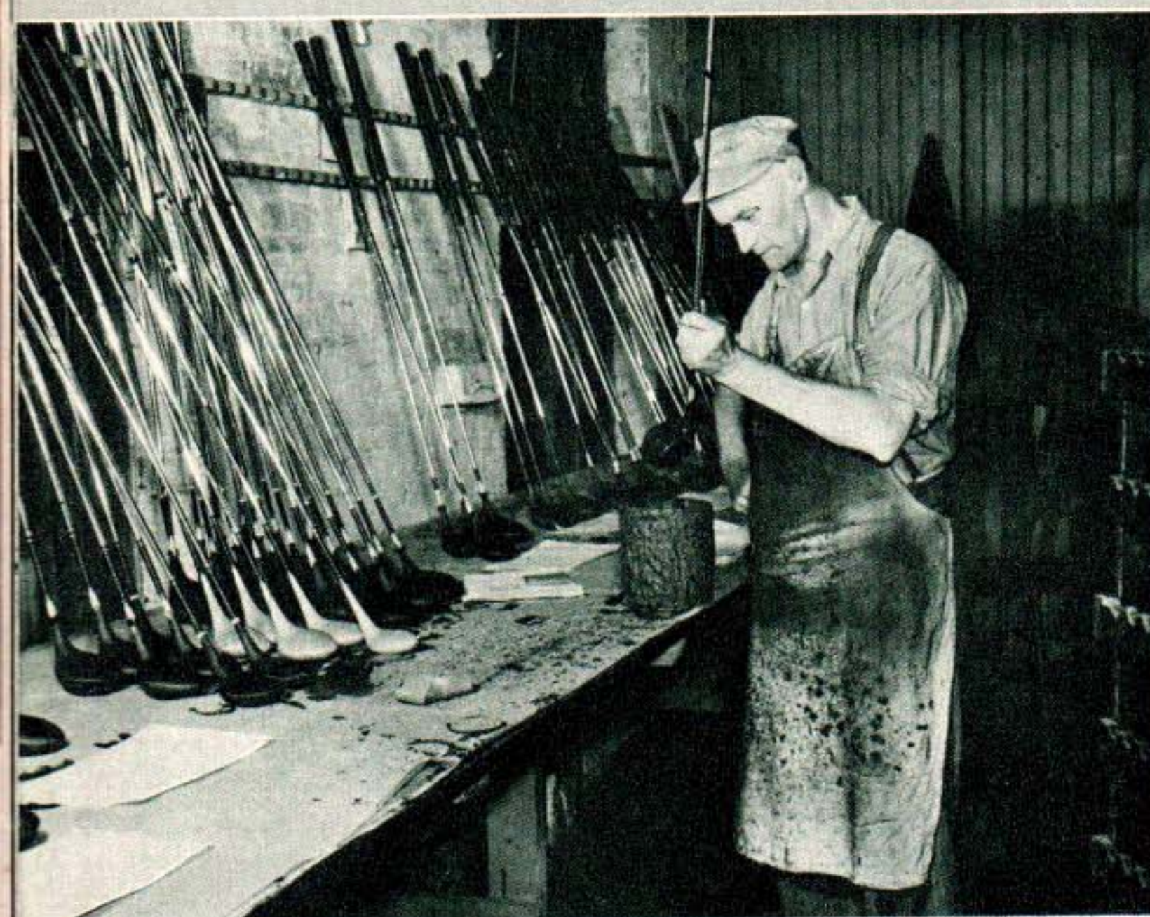
Finishing of golf club heads is the work of master craftsman at the big Hillerich and Bradsby plant
